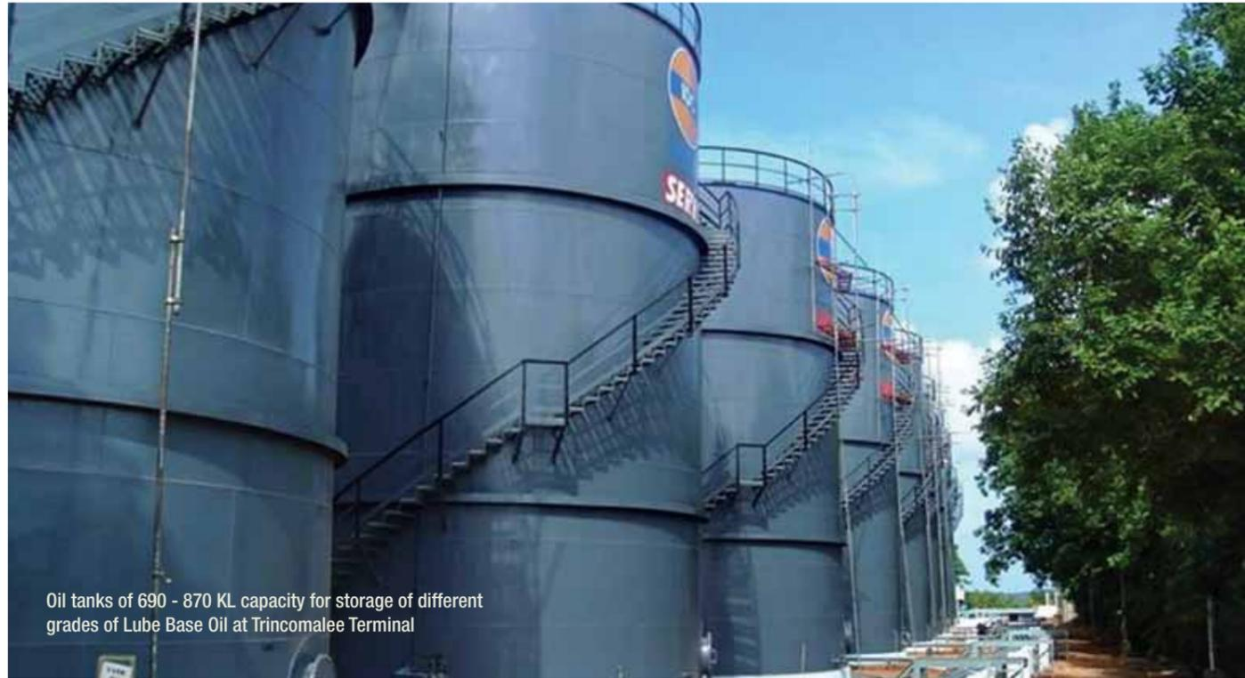
Oil tanks of 690 - 870 KL capacity for storage of different grades of Lube Base Oil at Trincomalee Terminal
