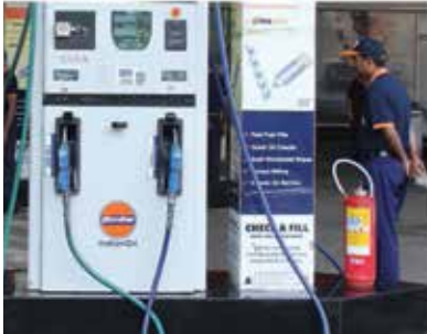
Two 10 kg / 9 kg DCP Fire Extinguishers are to be placed on each pump island.
