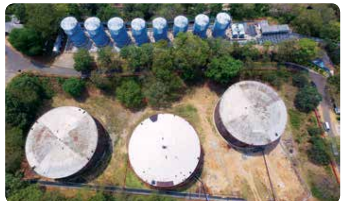
Facilities at Trincomalee Oil Terminal
