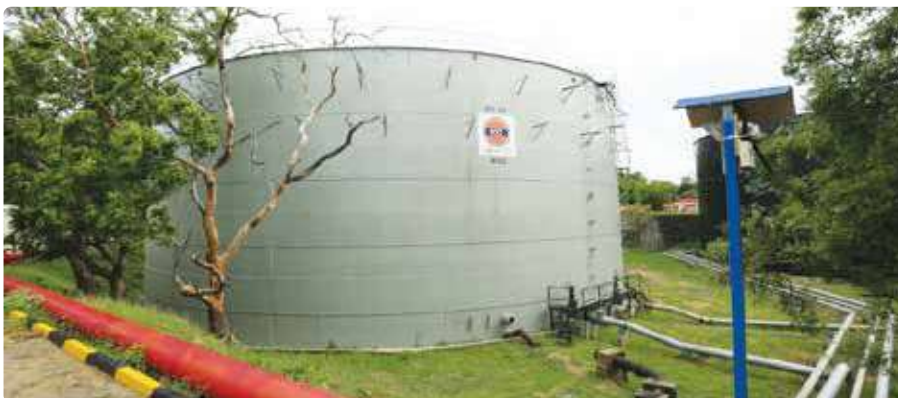
Storage Tank at Trincomalee
