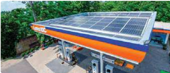
Revenue generation commenced of solar energy from canopy roof top panel at auto fuel stations.
